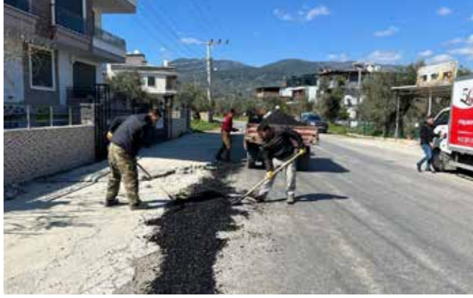
Tahtakuşlar Mah 25056 Sok Rothmix Yamalama
