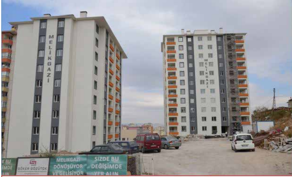
BATTALGAZİ MH. 2 BLOK 78 DAİRE
