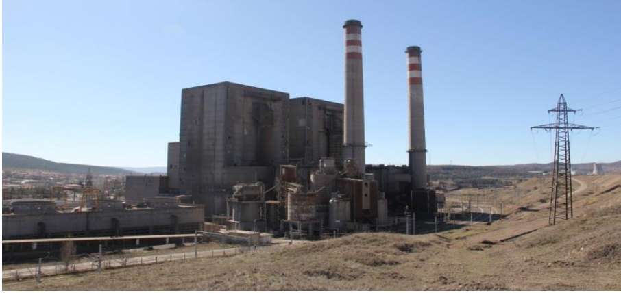
Tunçbilek Termik Santrali
