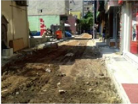
MURADIYE MAHALLESİ FIRIN SOKAK
