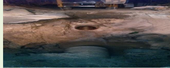
(İçme suyu asbest boru tamirati)
