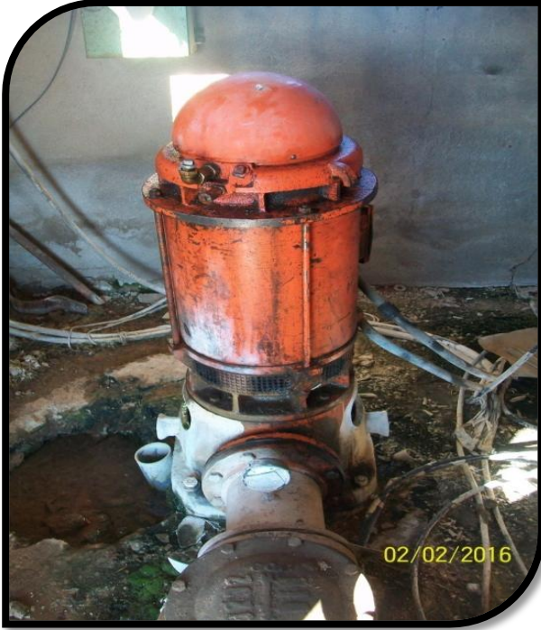
İnsuyu 1 nolu Pompa Yenilendi
