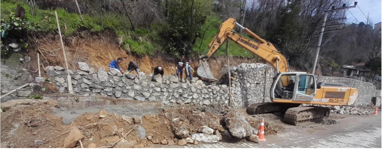
Mithatpaşa Dağyolu sokak
