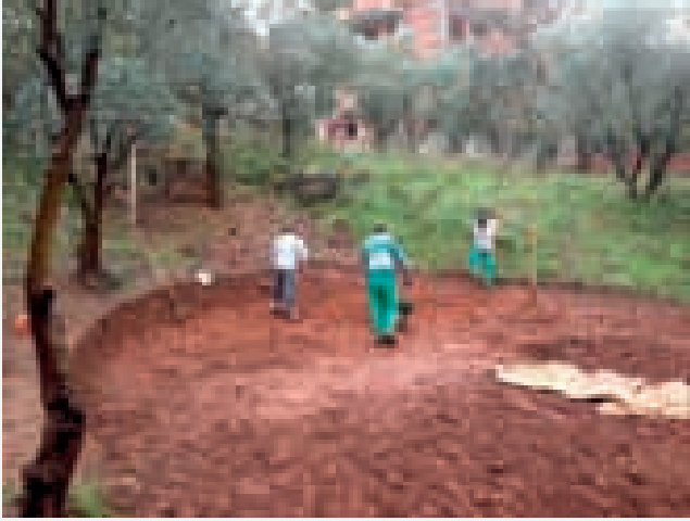
5-YENİMAHALLE RADAR CADDESİ PARK YAPIMI
