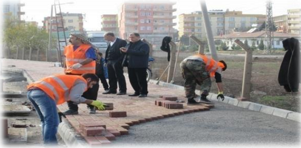
Viranşehir Beton Parke
