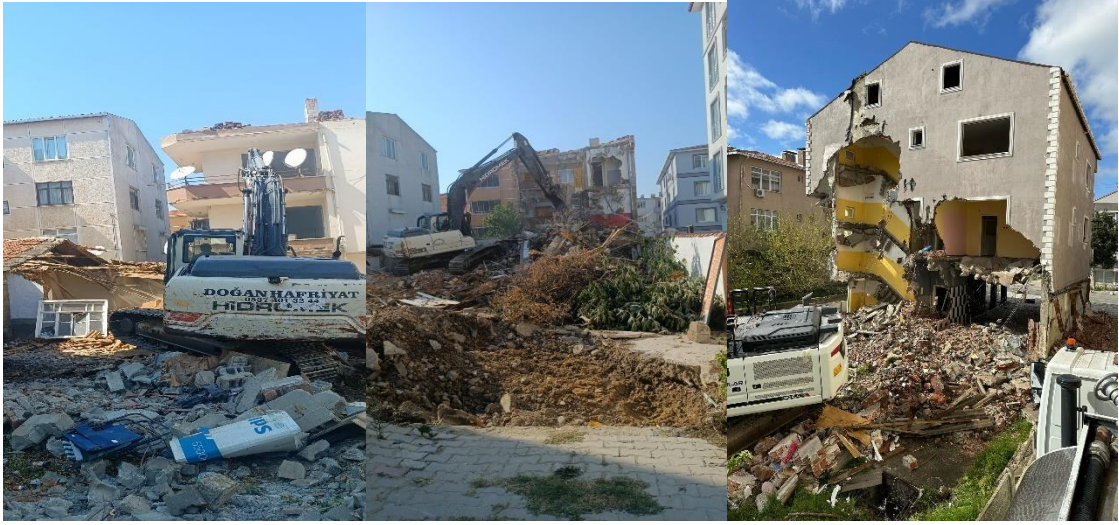
Kemalpaşa Mahallesi, Halim
