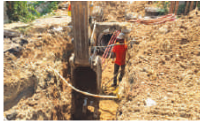
ORHANLI MAHALLESİ ANIT SOKAK
