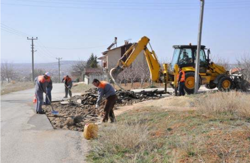
KERVANSARAY MAHALLESİ İMAMI AZAM CAMİİ CİVARI
