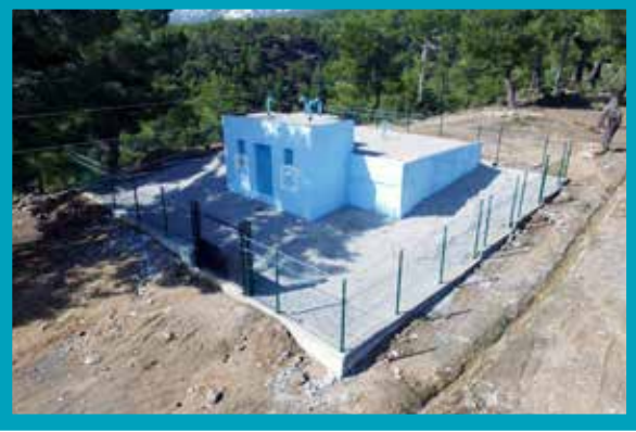
Acıpayam Akalan 2 Depo Yeni Hali
