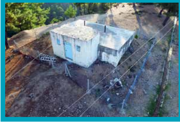
Acıpayam Akalan 2 Depo Eski Hali
