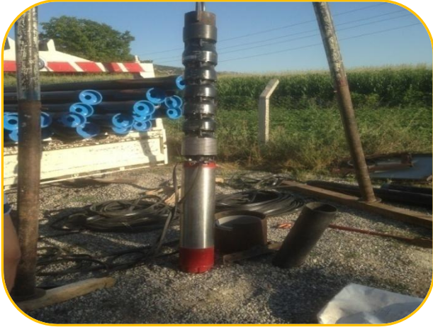
İnsuyu 1 Nolu Kuyu Yenilendi
