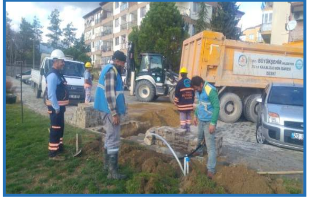
Karaman Mahallesi 1490/4 sokak park
